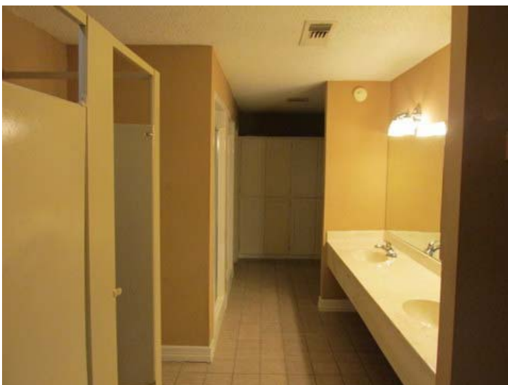
Clubhouse rest room
