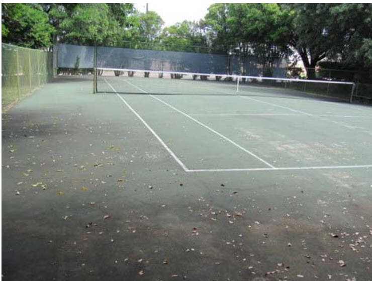
Tennis court overview
