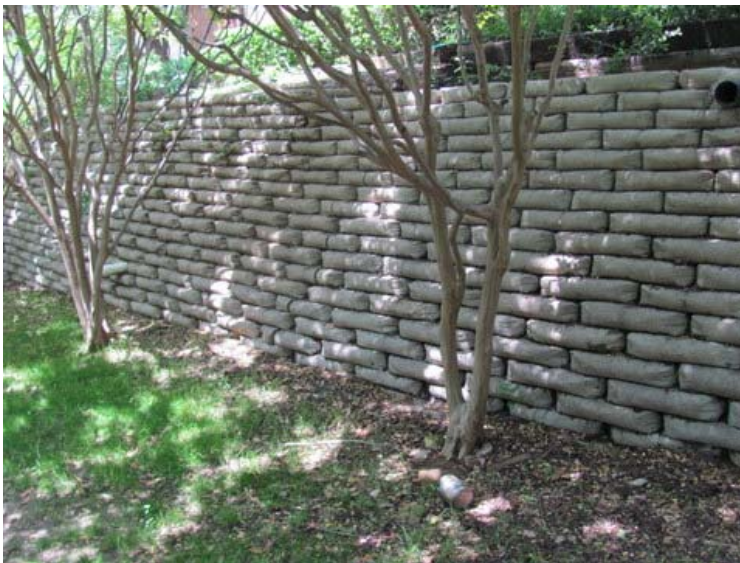
Concrete retaining wall
