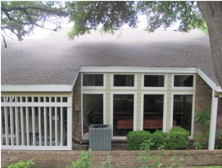
Clubhouse side overview
