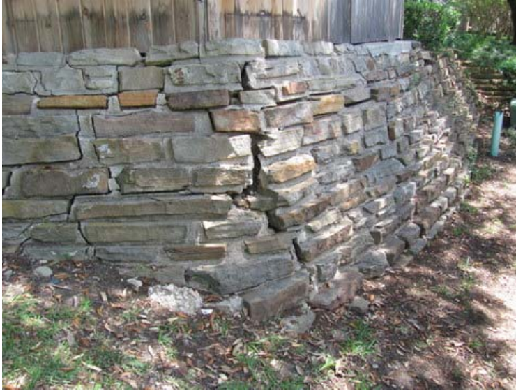
Masonry retaining wall
