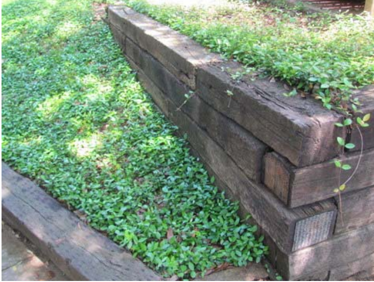
Timber retaining wall
