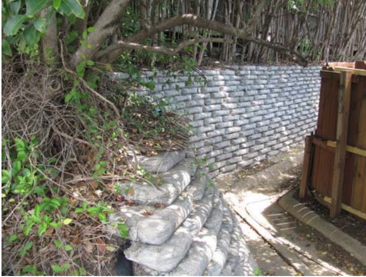
Concrete retaining wall
