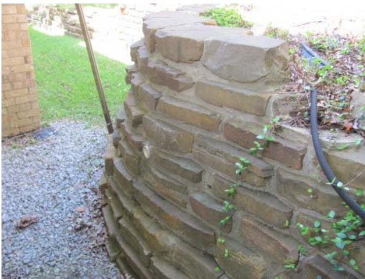
Masonry retaining wall
