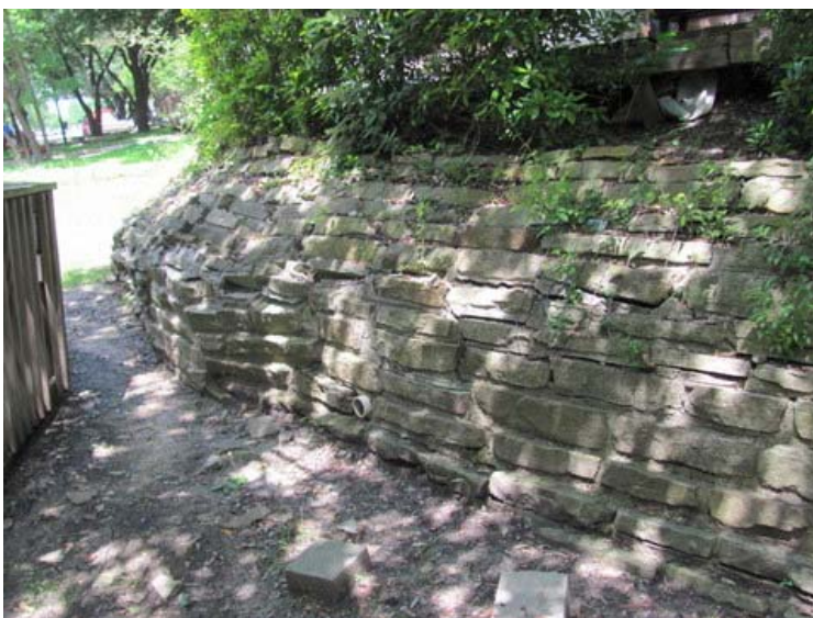
Masonry retaining wall
