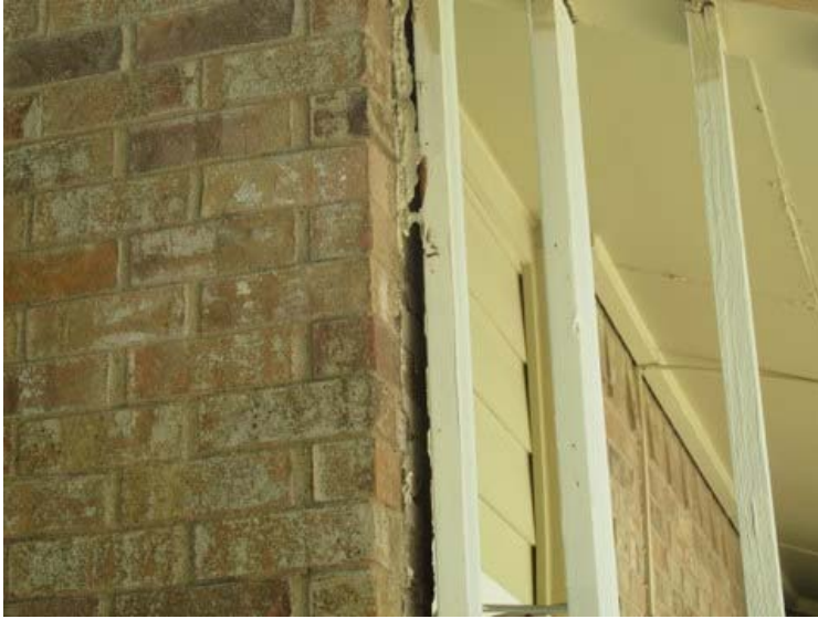
Wood siding at clubhouse
