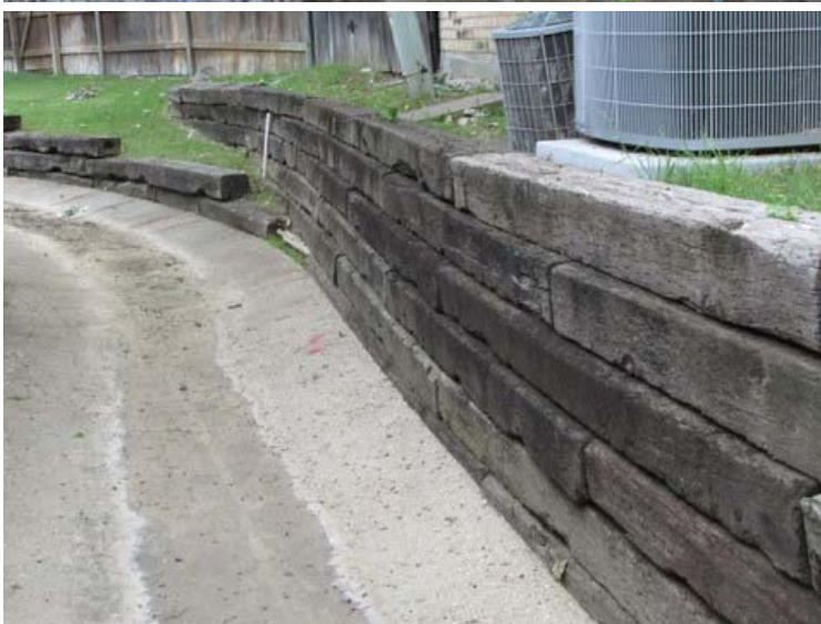
Timber retaining wall
